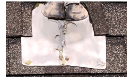
Damaged or aged roof jacks may allow water leaks in your roof.
