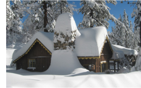
Heavy snow and ice damming can weigh down your roof potentially causing water leaks or worse.
