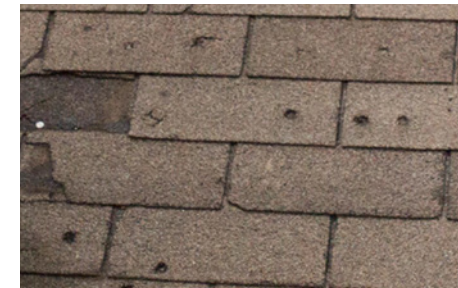
Large and fast-moving hail may compromise your roof structure's integrity.
